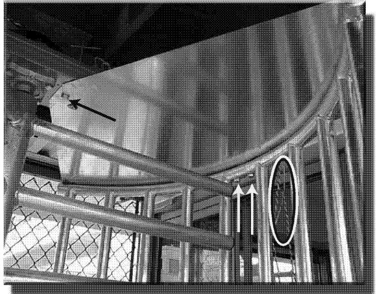
(Fig. 14) Mark and drill #10 pan head sheet metal screws. Yoke guard plate attached.
