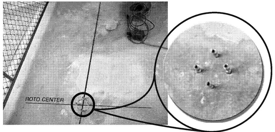
(Fig. 4) Anchors ready to be tapped into holes
